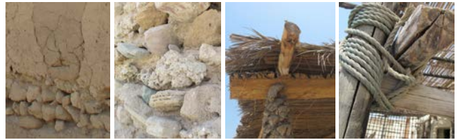
Figure 17. The materials used for the construction of a house with Badgir
