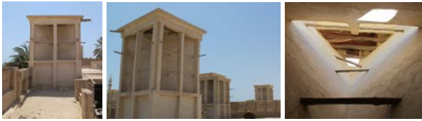
Figure 13. The Badgir and one of the ducts receiving winds
