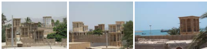
Figure 2. The wind towers of the city of Kong - The angle of Badgirs is inclined a few degrees to the prevailing wind
